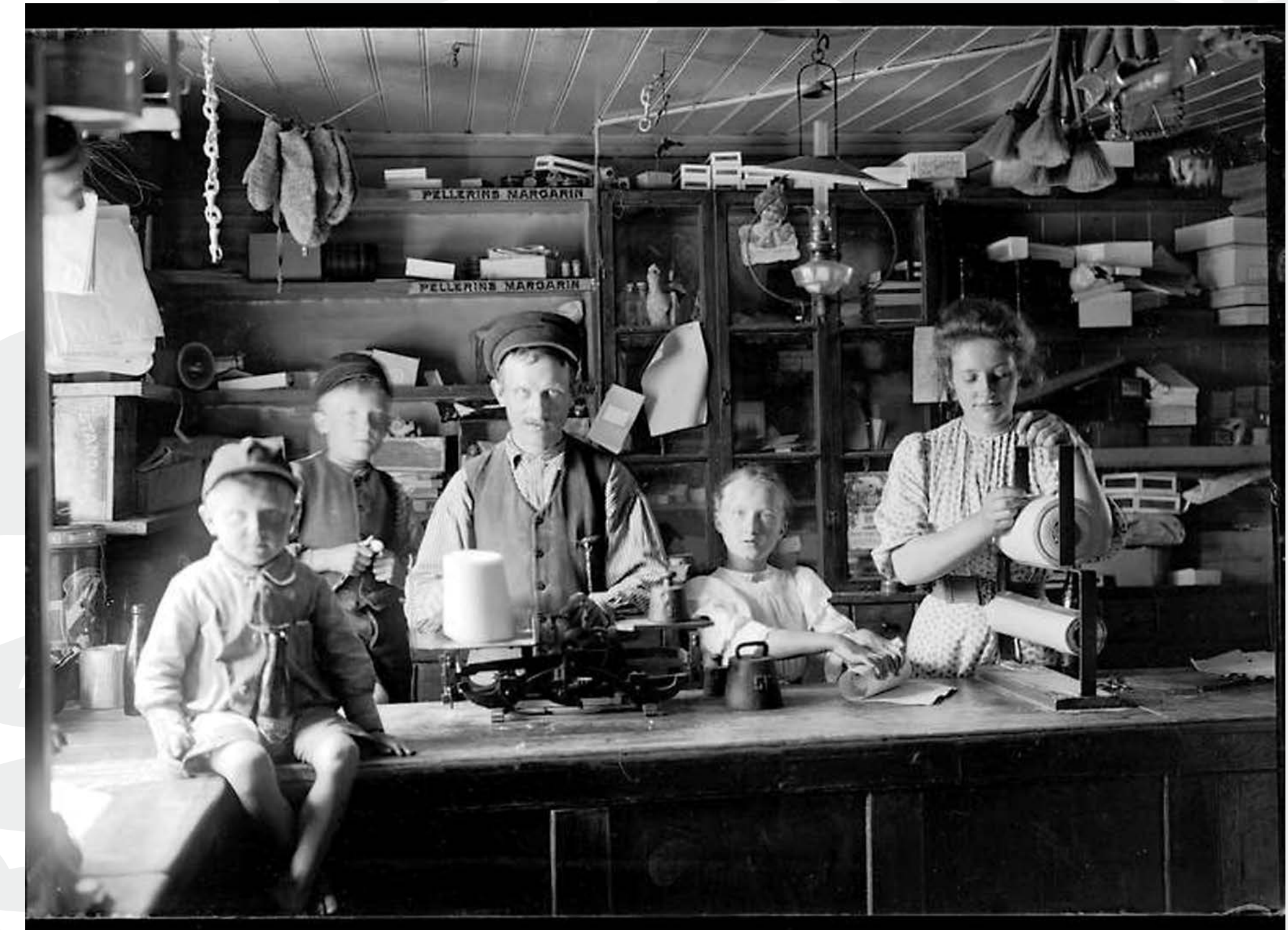
Operating a store was a family affair as you can see from this interior photo of the Ryberg family’s country store in Dalsland, ca 1895. Photo by Olof Jonsson, Courtesy of Vänersborgs Museum
